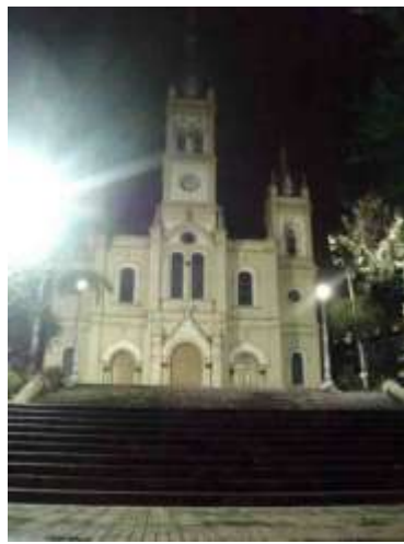
Sao Jose Church in Belo Horizonte.
